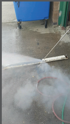
Paint Stripped from Cast Iron
